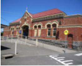
Ascot Vale Railway Station.JPG
