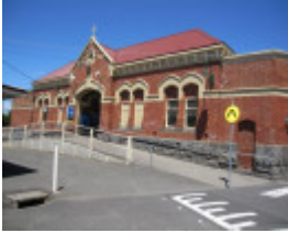
Ascot Vale Railway Station.JPG
