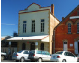
FORMER SHOP AND RESIDENCE SOHE 2008
