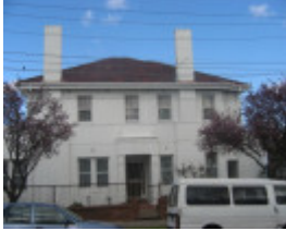
662 High Street, Reservoir
