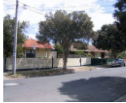
War Service House Commission 17,19 & 21 Arthur Street
