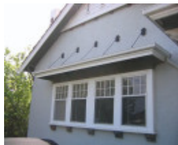
16 Spencer Street: Window and Hood Detail
