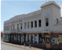
HO40 (1) - Rising Sun Hotel, 193 Geelong Road, Footscray.JPG
