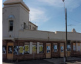
HO40 (2) - Rising Sun Hotel, 193 Geelong Road, Footscray.JPG
