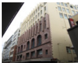
DJs former Coles_rear elevation_16 Jan 08
