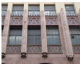
DJs former Coles_rear facade detail_16 Jan 08
