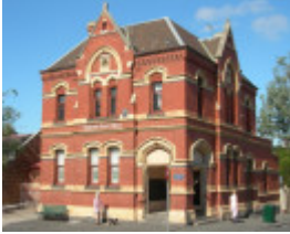
PARKVILLE POST OFFICE AND QUARTERS SOHE 2008
