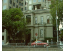
1 former residence 61 spring street july01
