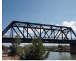
HO107(2) - Rail Bridge over Maribyrnong River & Tunnel, Bunbury Street, Footscray.JPG
