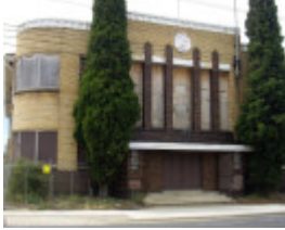
HO114 (3) - Olympic Tyre & Rubber, 56-84 Cross Street, West Footscray.JPG
