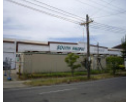
HO114 (2) - Olympic Tyre & Rubber, 56-84 Cross Street, West Footscray.JPG
