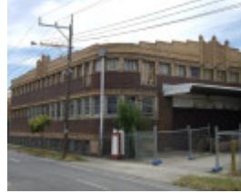
HO114 (1) - Olympic Tyre & Rubber, 56-84 Cross Street, West Footscray.JPG
