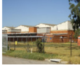
HO125 (3) - Bradmill 341-351 Francis Street, Yarraville.JPG
