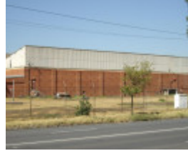
HO125 (1) - Bradmill 341-351 Francis Street, Yarraville.JPG
