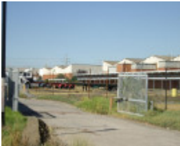
HO125 (4) - Bradmill 341-351 Francis Street, Yarraville.JPG
