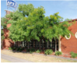
HO129 (1) - Hopkins Odlum, 268 Geelong Road, West Footscray.JPG
