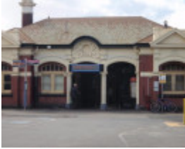
HO49(1) - Footscray Railway Station.JPG
