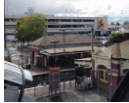
HO49(2) - Footscray Railway Station.JPG
