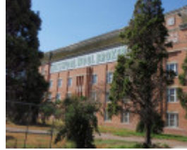
HO160 (2) - Australian Estate Wool Store, 47-61 Sunshine Road, West Footscray.JPG
