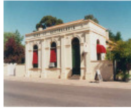
former bank of australasia conness street chiltern front view
