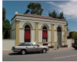
1 former bank of australasia conness street chiltern front view
