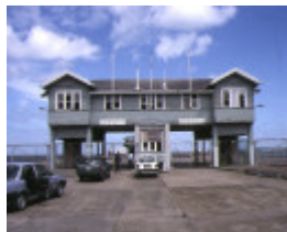
1 princes pier beach road port melbourne entry building front view
