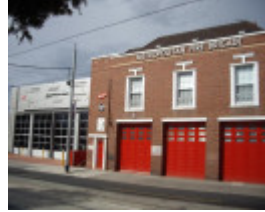
HO116 (2) - Footscray Fire Station Complex, 67-71 Droop Street, Footscray.JPG
