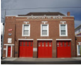
HO116 (1) - Footscray Fire Station Complex, 67-71 Droop Street, Footscray.JPG
