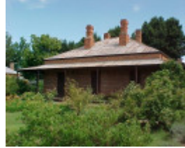
1 lakeview victoria street chiltern front elevation jan00
