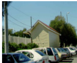
clayton railway station rear upside building sw nov1998
