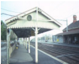
clifton hill railway station complex hoddle street clifton hill platform jun1984
