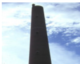
1 shot tower alexandra parade clifton hill tower view
