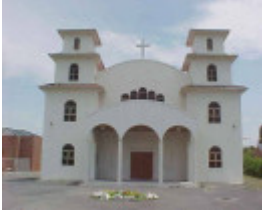
View from Amis Crescent
