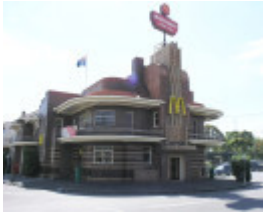
FORMER UNITED KINGDOM HOTEL SOHE 2008
