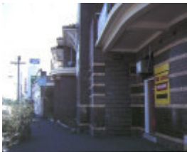
former united kingdom hotel queens parade clifton hill view from street level dec1987
