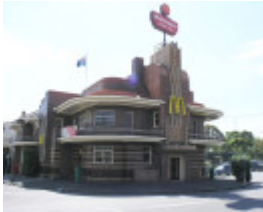
FORMER UNITED KINGDOM HOTEL SOHE 2008
