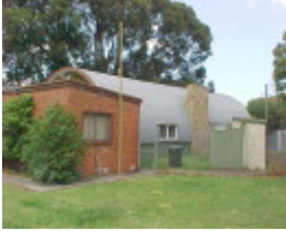
View of building from north-west
