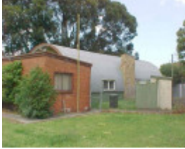
View of building from north-west
