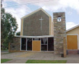
View of church from James Street
