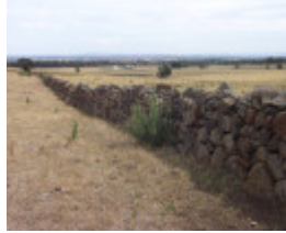
Dry Stone Wall R300
