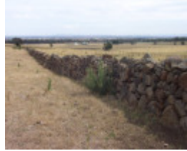
Dry Stone Wall R300
