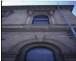
clunes post office detail exterior windows nov1984
