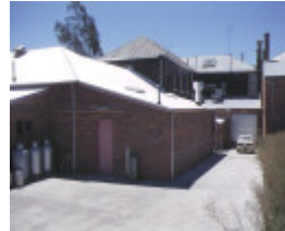
club hotel clunes rear view feb1991
