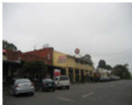
Railway Hotel Former Bunyip
