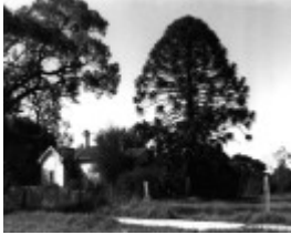
Beaconsfield Station Masters Residence Bunya Bunya
