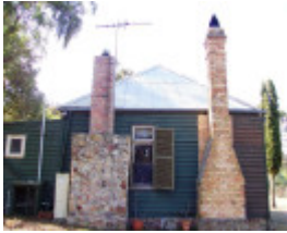
Paine's Cottage Chimneys
