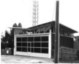
Bunyip Fire Station
