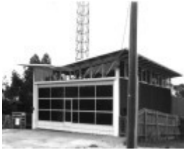
Bunyip Fire Station
