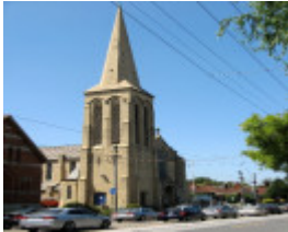
H2158 St Mark s Church from Burke Rd
