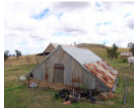
Underground water tank
