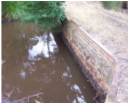
Finely constructed dam wall
