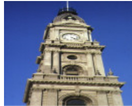
collingwood town hall clock tower detail jul1983
