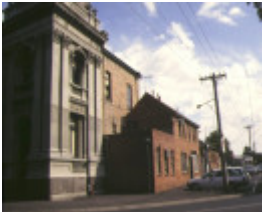
collingwood town hall rear view jul1983
