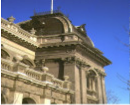
collingwood town hall balcony detail jul1983
