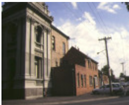
collingwood town hall rear view jul1983
