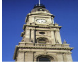
collingwood town hall clock tower detail jul1983
