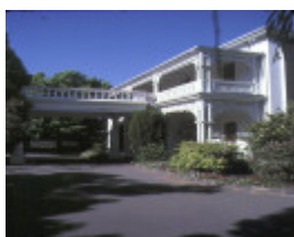
armadale house kooyong road armadale entrance jan1985
