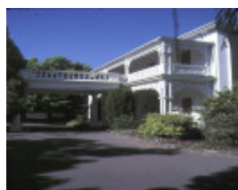
armadale house kooyong road armadale entrance jan1985
