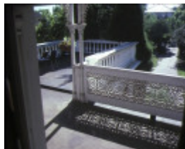
armadale house kooyong road armadale balcony jan1985
