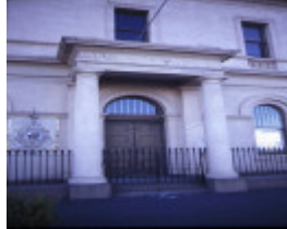
1 former es&a bank clunes front entrance
