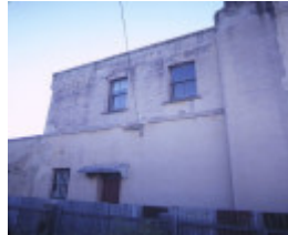
former es&a bank clunes back windows
