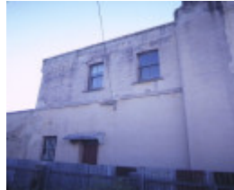
former es&a bank clunes back windows
