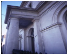
former es&a bank clunes front columns
