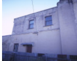
former es&a bank clunes back windows
