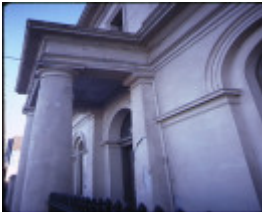
former es&a bank clunes front columns
