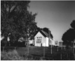
Elms & Iona State School SS3201 Site
