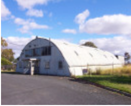
Former Army Radio Station
