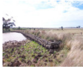
Former Clarke Dam
