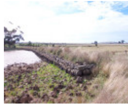
Former Clarke Dam
