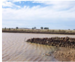
Former Clarke Dam
