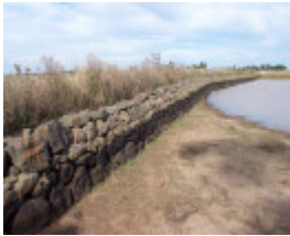
Former Clarke Dam
