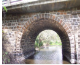
Bridge over the Kororoit Creek
