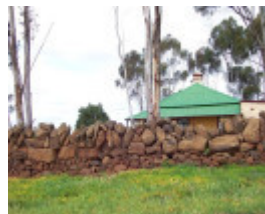
Dry Stone Wall A272
