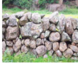
Dry Stone Wall A276
