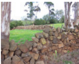
Dry Stone Wall A273
