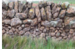
Dry Stone Wall A277
