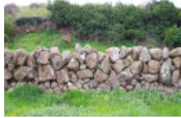
Dry Stone Wall A276
