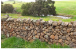
Dry Stone Wall A275
