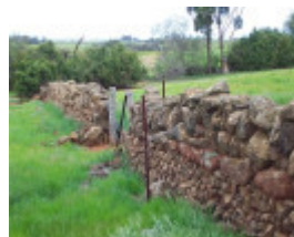
Dry Stone Wall A273
