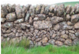
Dry Stone Wall A277
