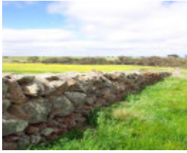
Dry Stone Wall A274
