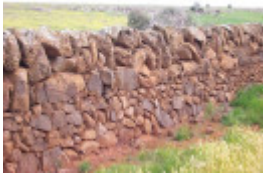
Dry Stone Wall A277
