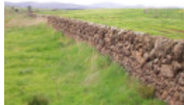
Dry Stone Wall A277
