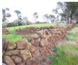
Dry Stone Wall A272
