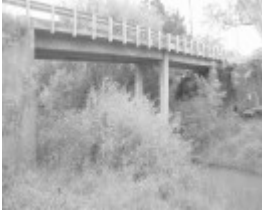
Bridge Road bridge over the Toolern Creek
