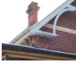
Kippenross - eave detail
