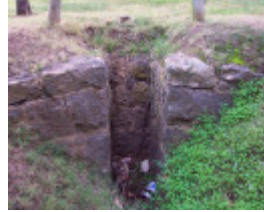
Stonework beside the Toolern Creek. This secured a pipe which supplied water to the reservoir from a small dam on the creek
