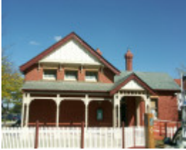
Former Melton Courthouse
