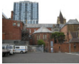
Francis Ormond Bldg_Melbourne_rear view_8 Jan 2008
