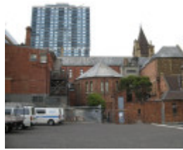
Francis Ormond Bldg_Melbourne_rear view_8 Jan 2008
