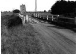
Swamp Bridges & Swamp Drains
